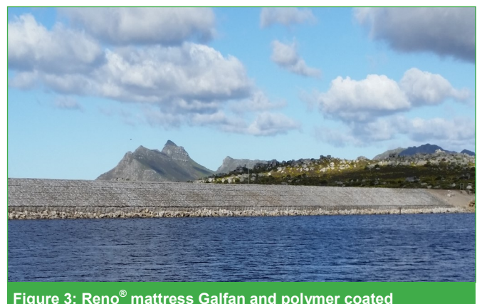
Figure 3: Reno ® mattress Galfan and polymer coated
