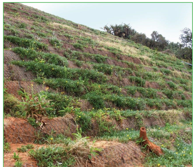
Figure 3: Green Terramesh® Galfan Polymer coated
