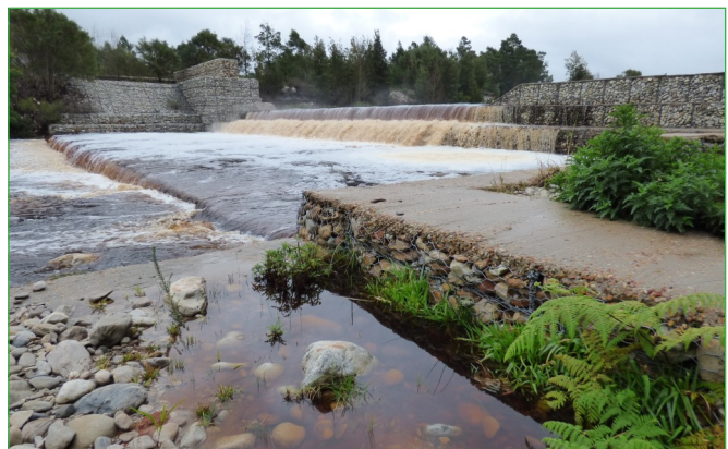
Figure 3: Gabions Galfan (Zn 95Al5) & Polymer coated
